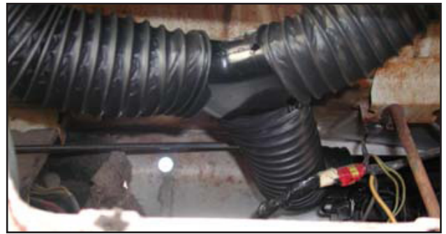
Photo 11 - Connect Defrost Outlets
