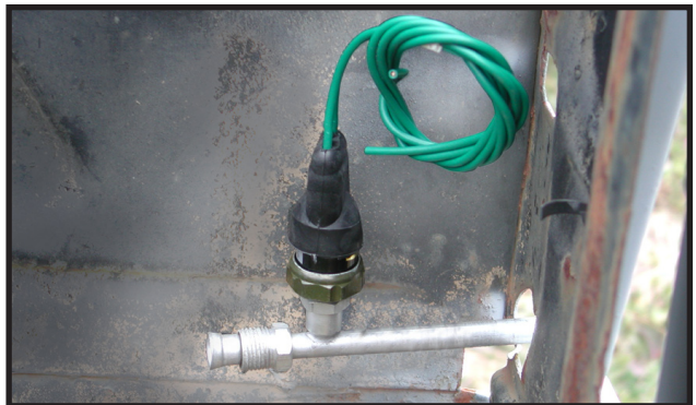
Photo 22 - Install Safety Pressure Switch
