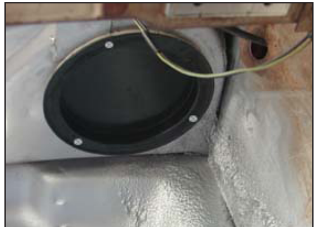
Photo 1 - Install Fresh Air Block-off
