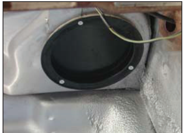
Photo 1 - Install Fresh Air Block-off
